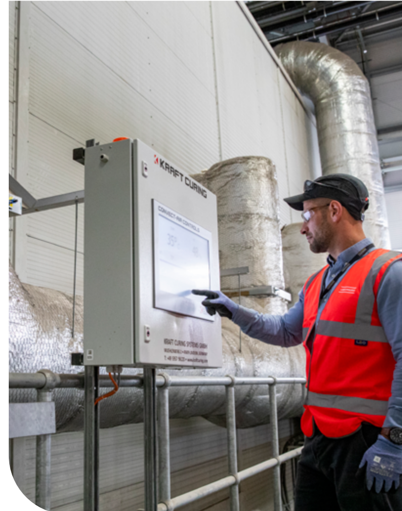
Image: New electric ovens to support curing of low carbon concrete at our Centre of Excellence for Modern Construction, UK
