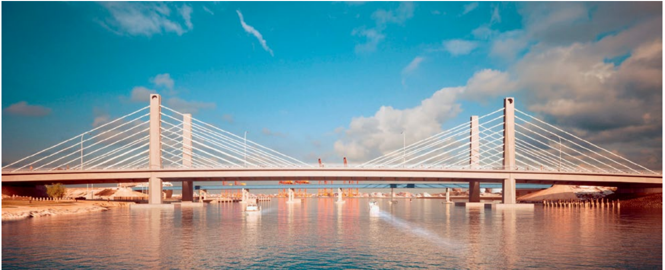
Image: Swan River Crossings Project – Fremantle Traffic Bridge, Perth, Australia
