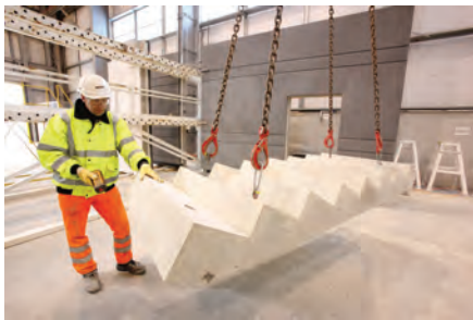
ABOVE: Views inside Laing O'Rourke's Centre of Excellence for Modern Construction (CEMC), Nottinghamshire.
