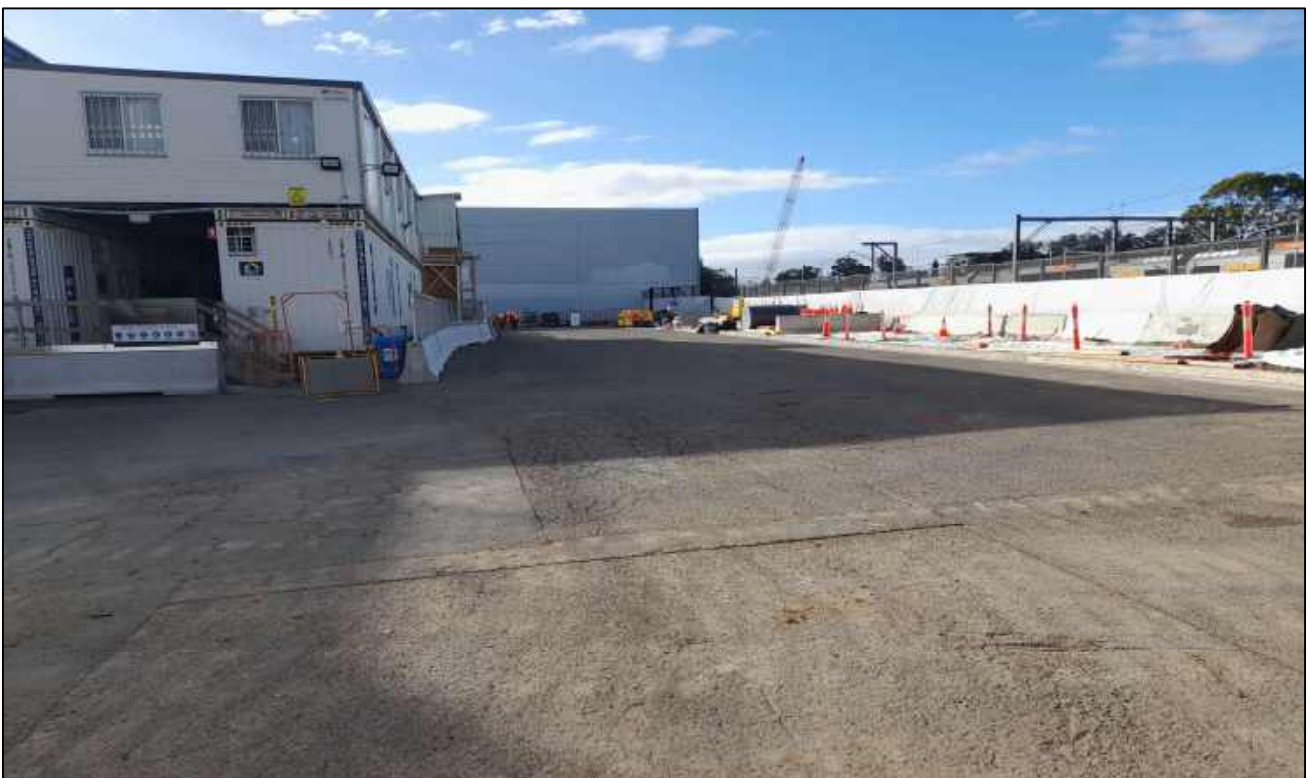
Photograph 2: Subject area (facing east). Date: 10 April 2023.
